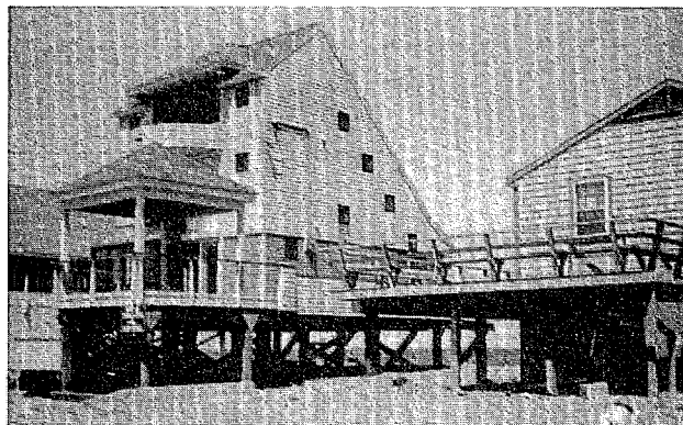
Residences are typically elevated on pressure-treated, cross-braced wood piles. One local contractor constructs over 25 residential elevation projects a year.
