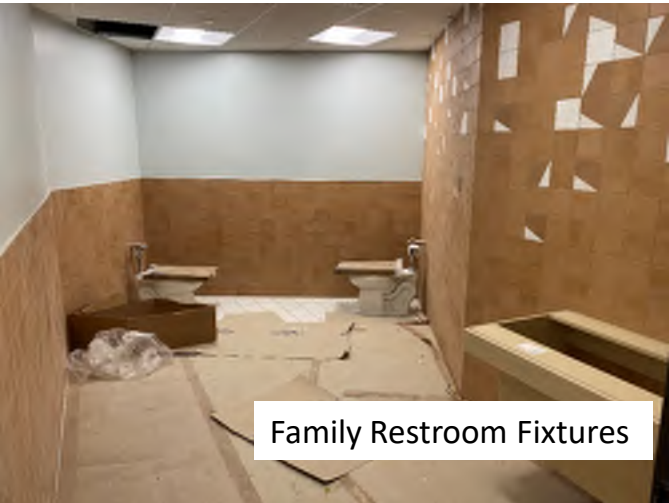
First Floor Addition Creation Station and Makers Space
